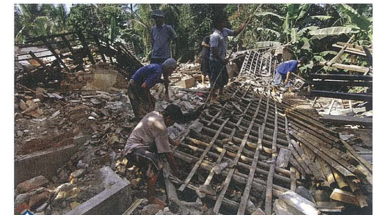
E Collapsed buildings in Yogyakarta
